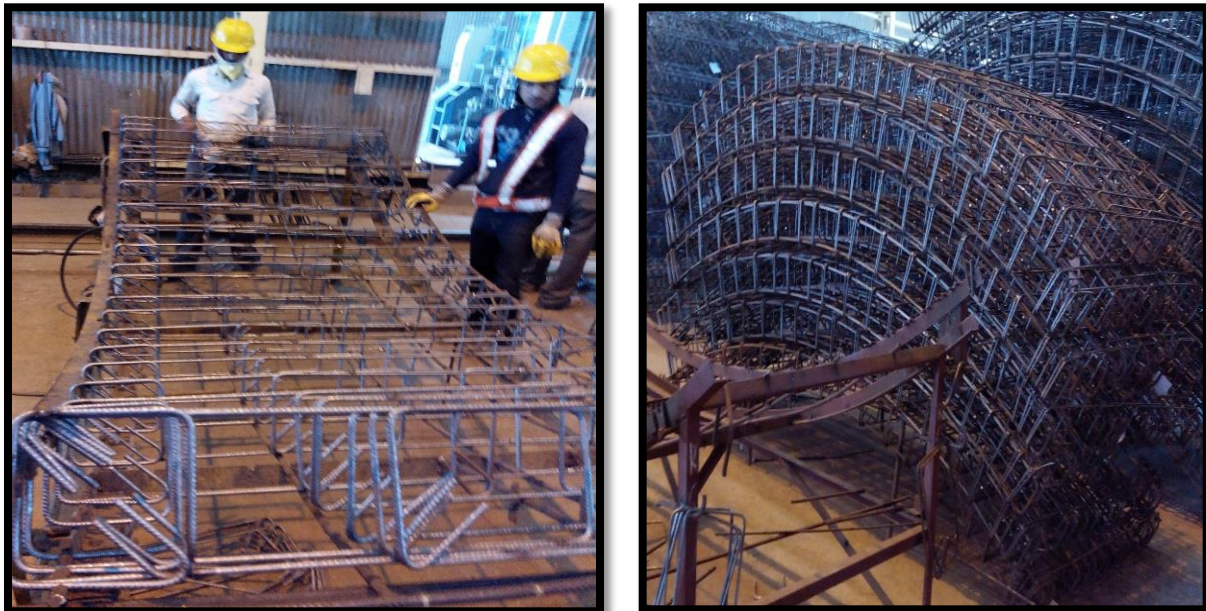
Figure 3: Reinforcement in a jig machine (L) and reinforcement cage for tunnel segments (R)
