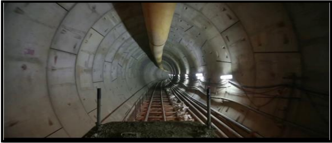
Figure 6: Assembled tunnel segments in a tunnel.
