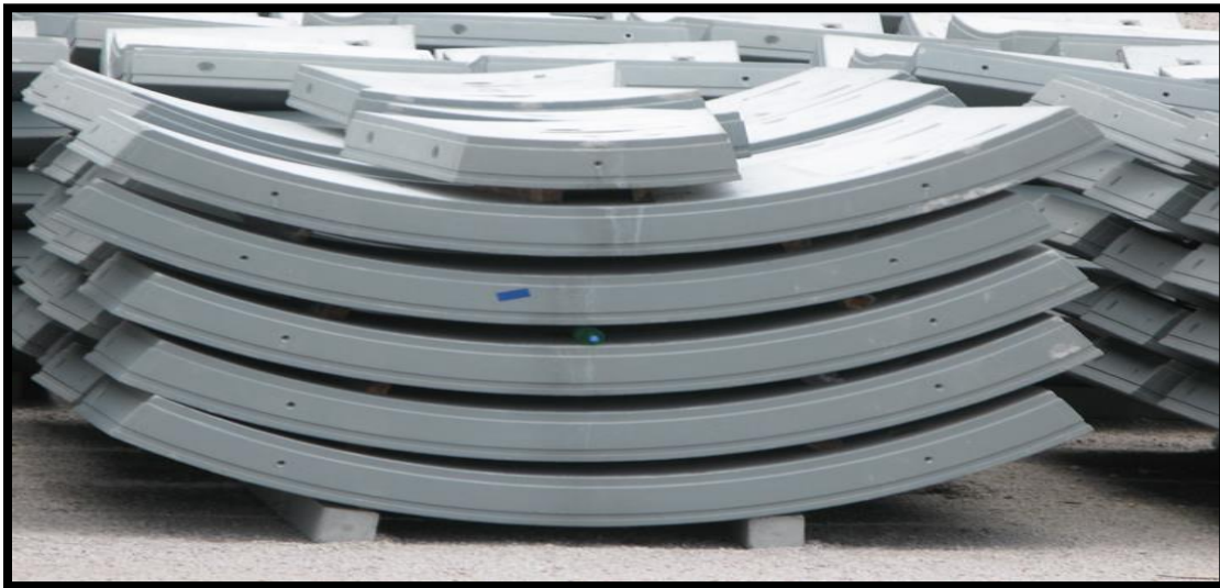
Figure 5: Storage of concrete segments
